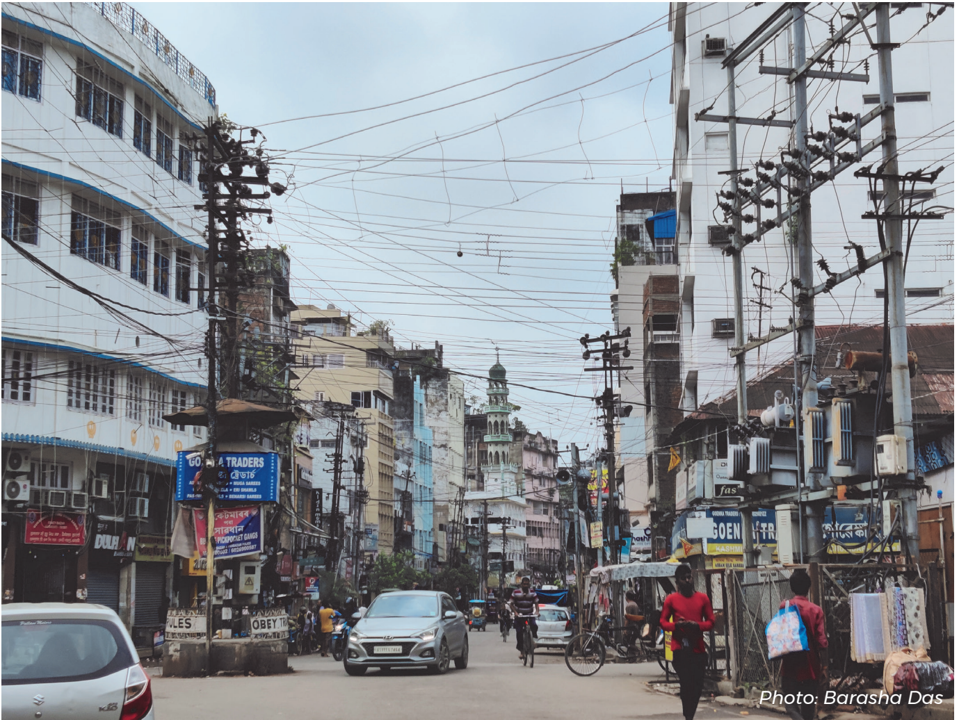
Fancy Bazaar area of Guwahati is cluttered with buildings
