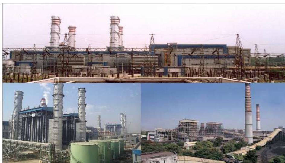
Figure 3: Thermal Power Plants
